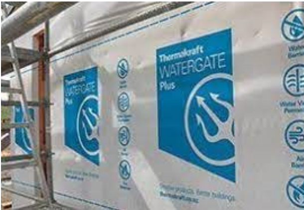
DIAGRAM 4 – leave openings covered
