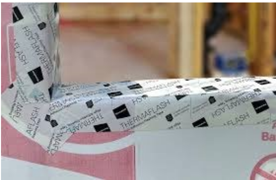
DIAGRAM 7 – bottom butterfly strip
